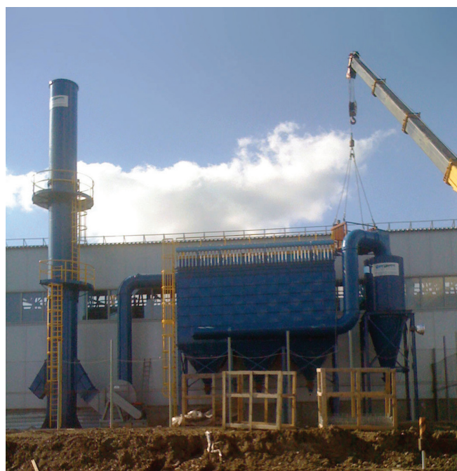
■ Suction and filtration system for dusts from grinding, flow rate 25,000 m 3 /h - Ukraine
