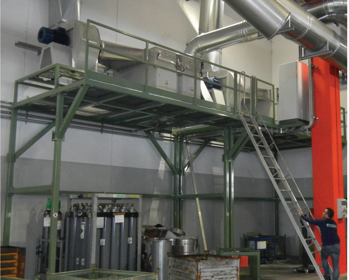
ENERPRESS filters on independent supporting structures dedicated to die casting machines with fans and expulsion chimneys. Italy
