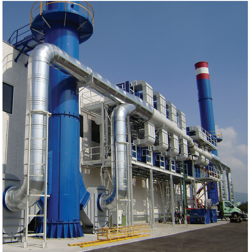
ENERPROG centralized suction and filtration system in 12 modules for a total suction flow of 200,000 m 3 /h dedicated to 22 presses - Italy
