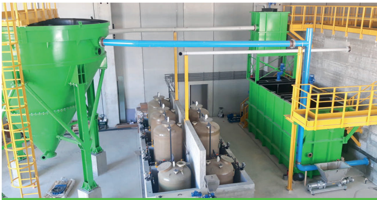
■ Soil washing plant, including steel structures, piping and installation – Italy
