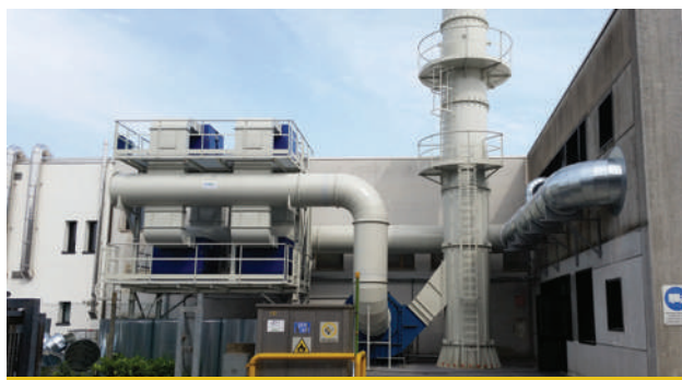
ENERPROG centralized suction and filtration system in 4 modules dedicated to 7 presses – Italy
