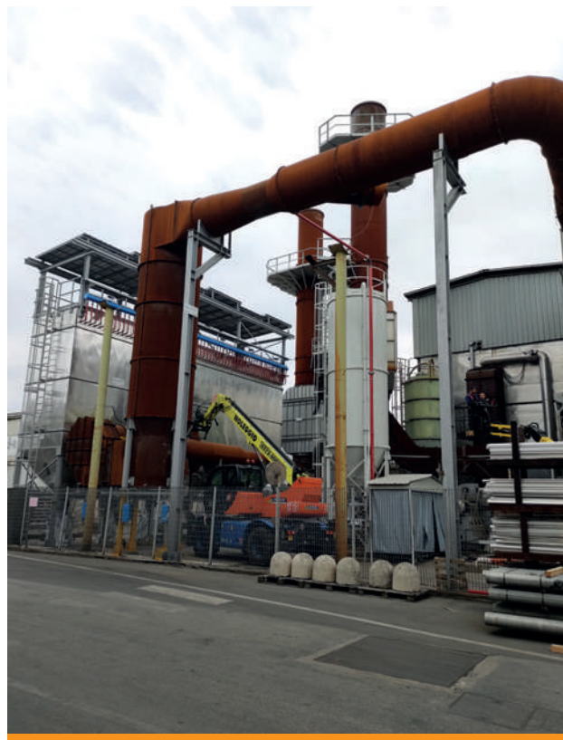
■ Aspiration and filtration plant for aluminium melting furnace with double chamber, complete with chemical inertisation system through storage, dosing and dry injection of reagent.
