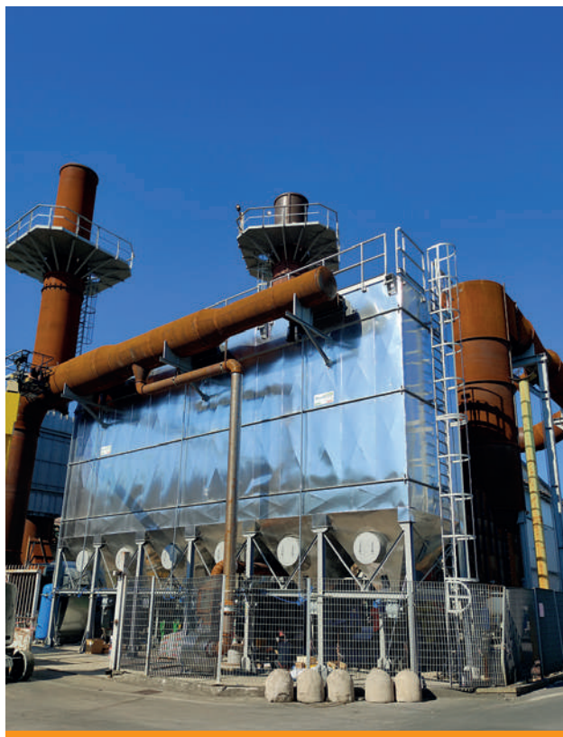
■ Aspiration and filtration plant for aluminium melting furnace with double chamber, complete with chemical inertisation system through storage, dosing and dry injection of reagent.
