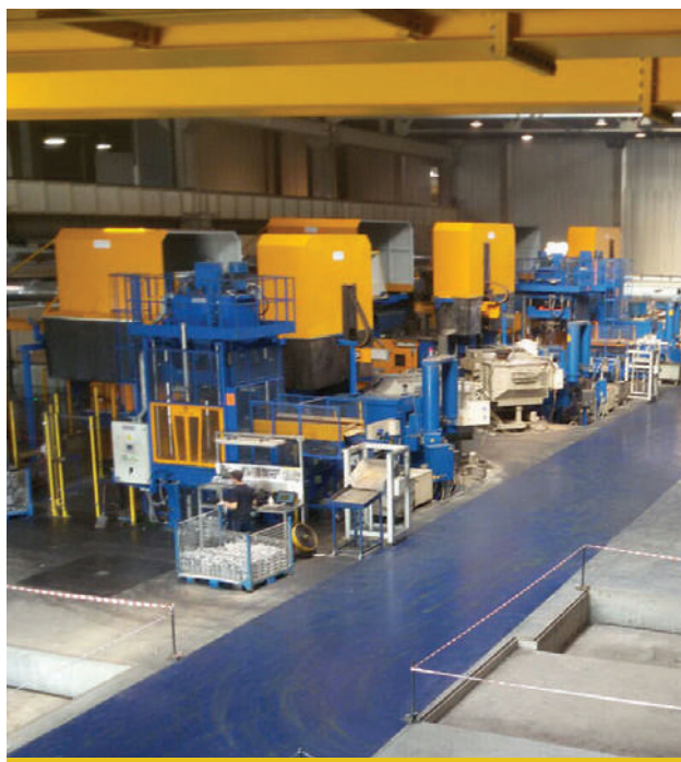
Hoods into two parts on COLOSIO PFO die-casting machines of different tonnages connected to a centralized suction and filtration system ENERPROG. Russia
